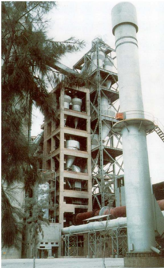
Figure 2: The modernised production line with the new PYROCLON® calciner on the left and existing raw-mix silo plant in front.
