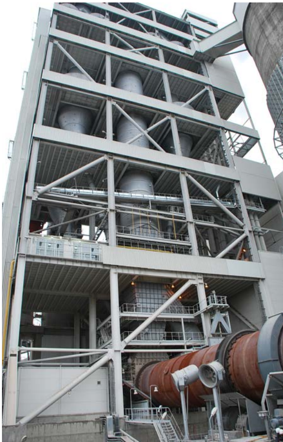
Figure 1. Dry process cement production line at the Pervomaysky plant.
